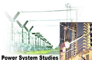
Power System Studies
